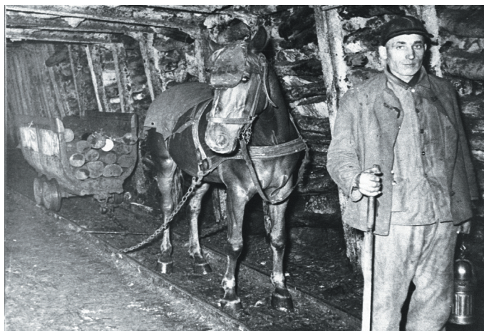
Ryc. 4. Transport materiałów do przodka (Gisman, 1950)
